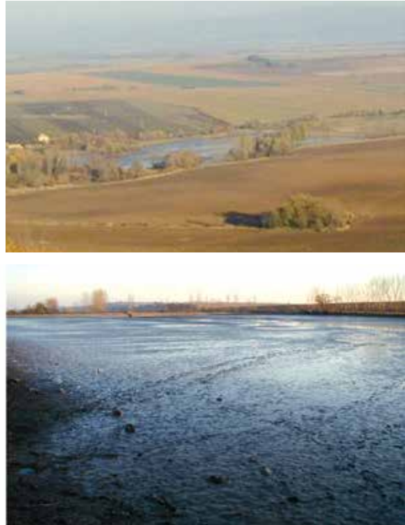
Figure 14.10. Top: A sediment control basin in a Central European landscape where conventional tillage is widely used. Bottom: Sediment regularly fills the basin and needs to be dredged.
