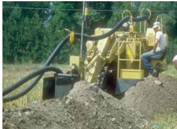
Figure 17.13. Left: Drainage ditch removes excess water and lowers water table. Right: Installation of perforated corrugated PVC drain lines using a laser-guided trencher.
